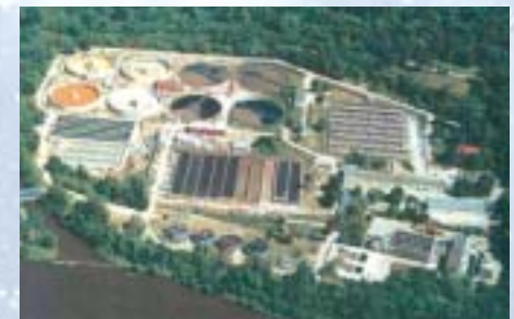
Waste water treatment plant
